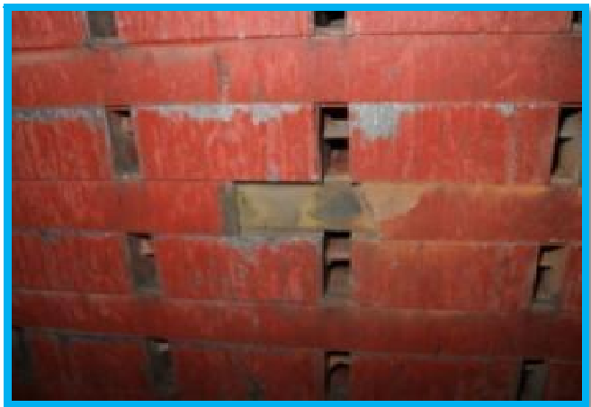
Photograph 2: Broken Wedge
