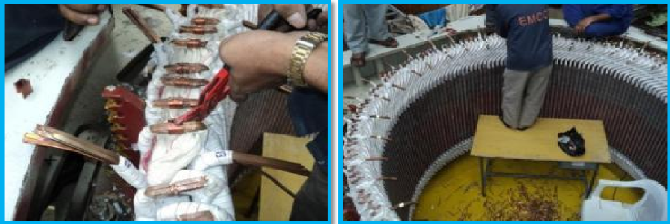
Photograph 18: Stator Coil Rewinding works
