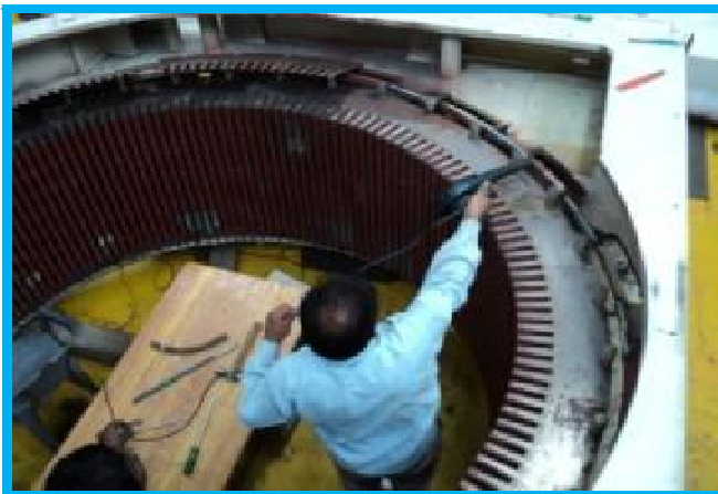
Photograph 15: Core Repair Works
