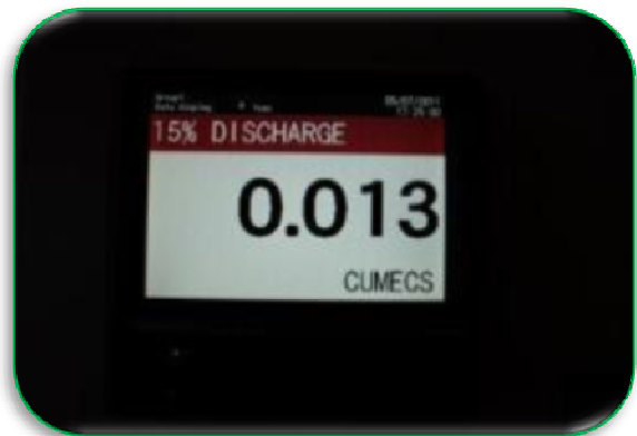
Display of the flow measuring device
