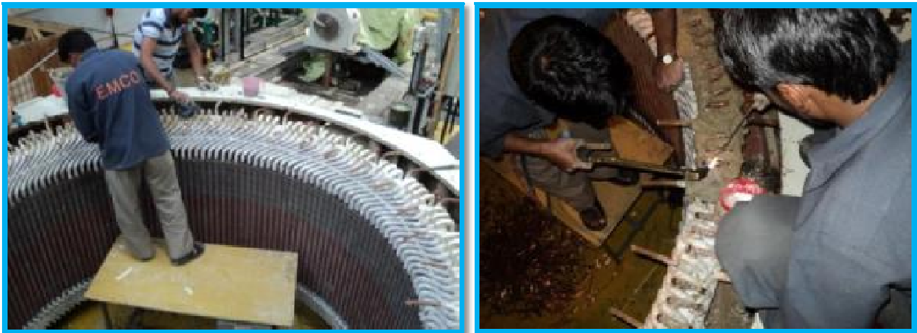
Photograph 17: Stator Coil Rewinding works
