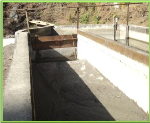
Choked silt flushing duct
