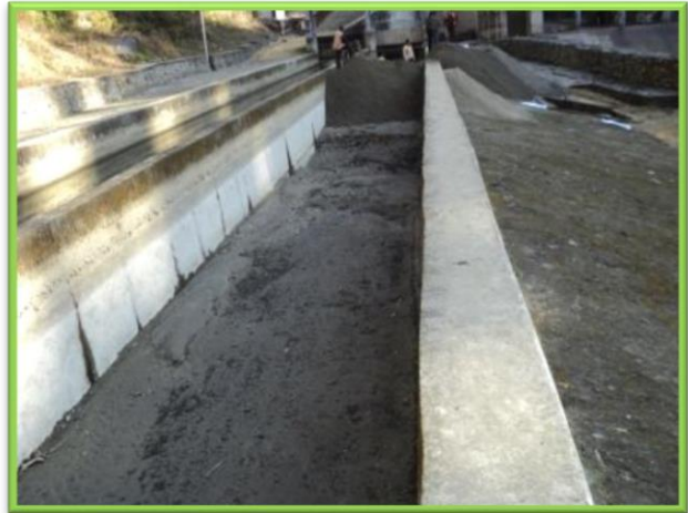
Choked silt flushing duct
