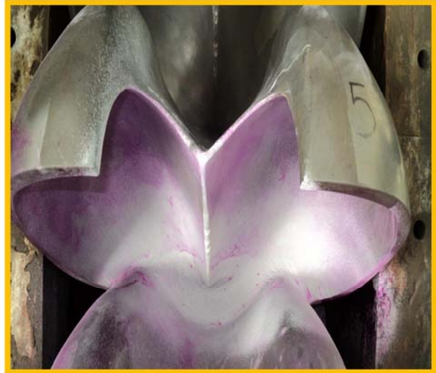
Repair work on the runner of Unit-II
