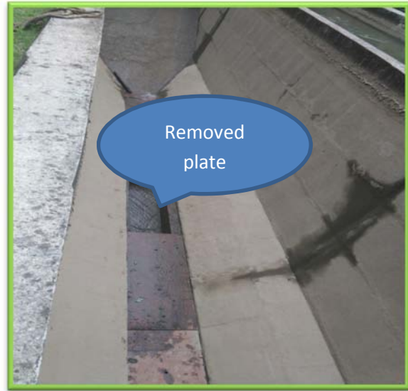
Removal of plates from alternate holes
