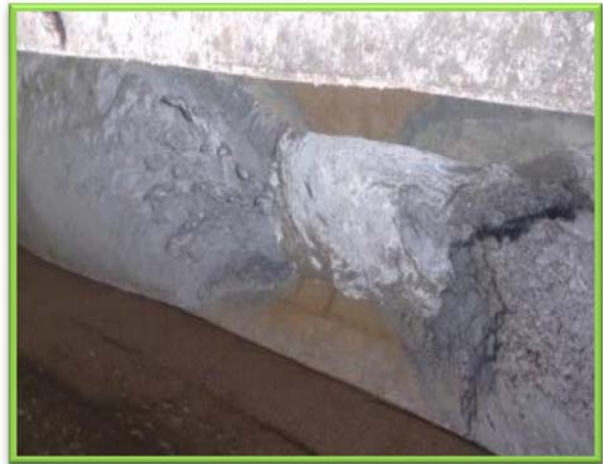
Completely choked silt flushing duct
