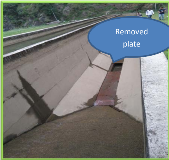
Removal of plates from alternate holes
