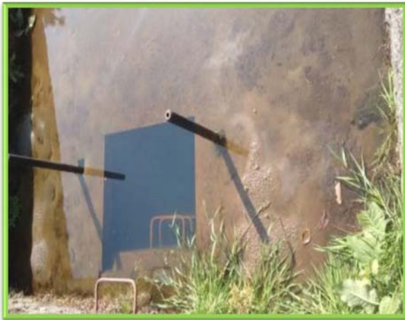
Completely choked silt flushing duct
