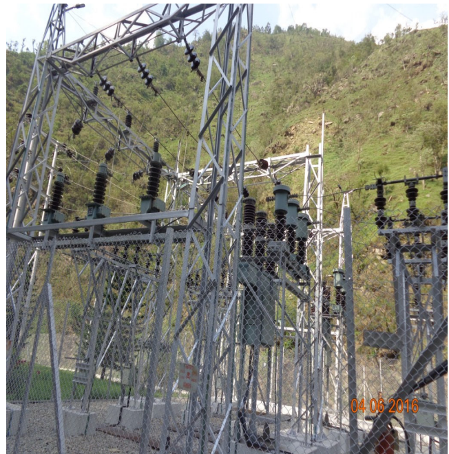
Fig.4.4 Painting of 33KV Switchyard
