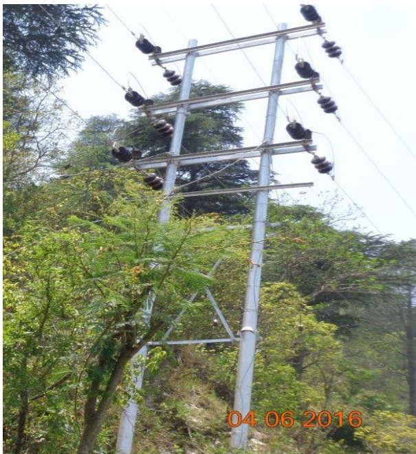
Fig. 4.3 Painting of Transmission line poles
