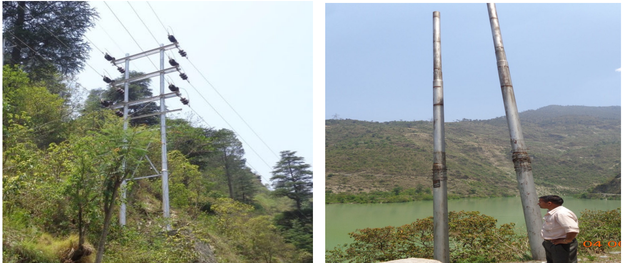
Fig. 4.8 Shifting of transmission line over newly erected pole
