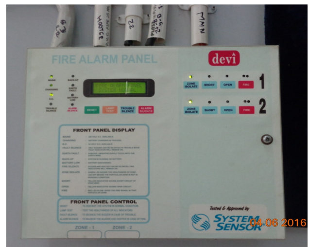
Fig. 4.7 Fire Alarm system in Control room
