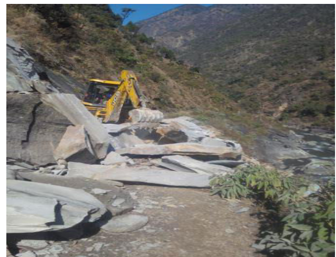
Fig.6.2 Restorations works carrying out
