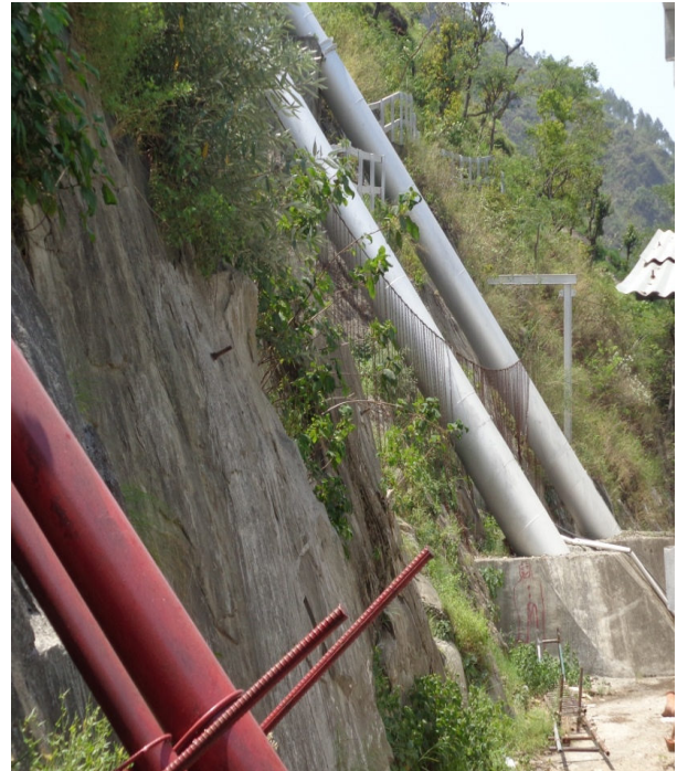
Fig.4.2 Painting of Penstock
