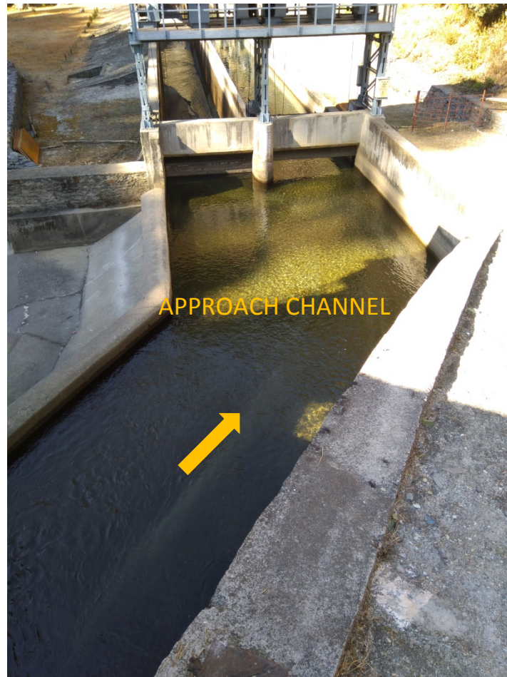
Approach Condition at the Inlet of Desilting Chamber
