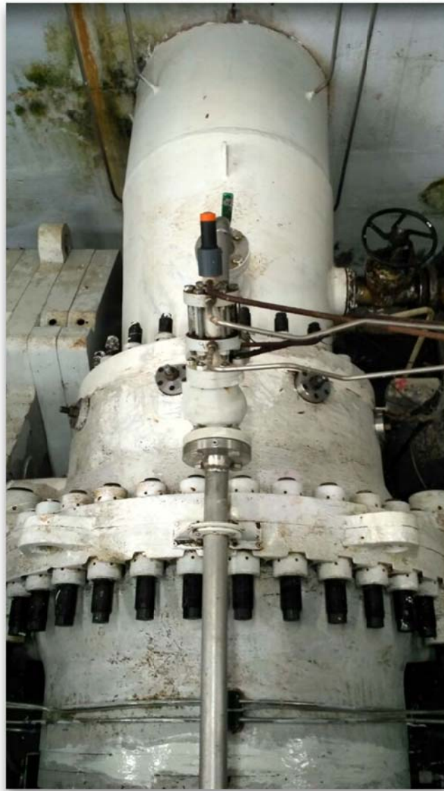
Penstock after Application Anti Rust Paint
