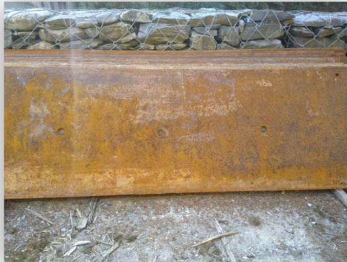
Steel Plates of Desilting Chamber
